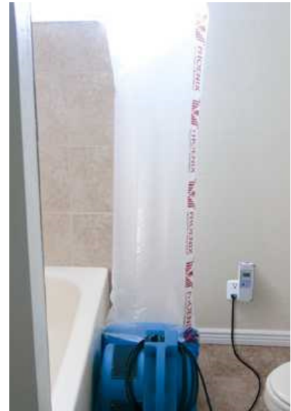
Air mover with ducting connected to Exhaust Controller
