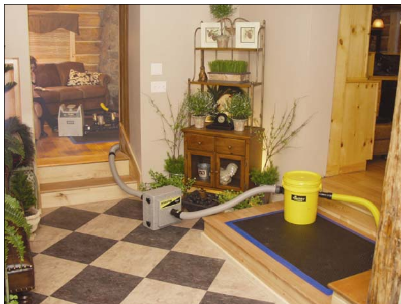
Vacuum drying and the use of HEPA Filtering systems, allows homes and businesses to be used during a dryout. (Large Single Port Panels shown)
